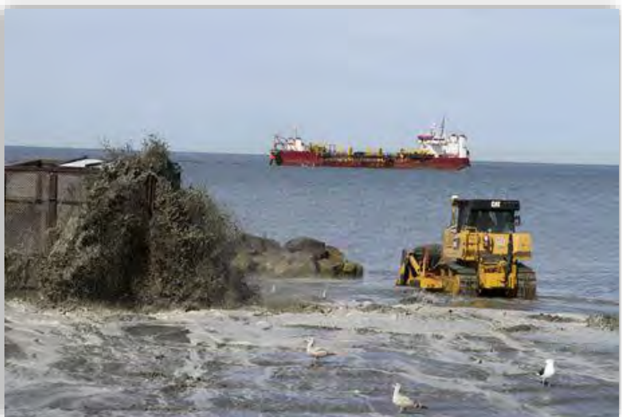
Figure 51 JBLE dredges the outfall of Skiffe's Creek to the James River on a regular basis to maintain training operations and access.
